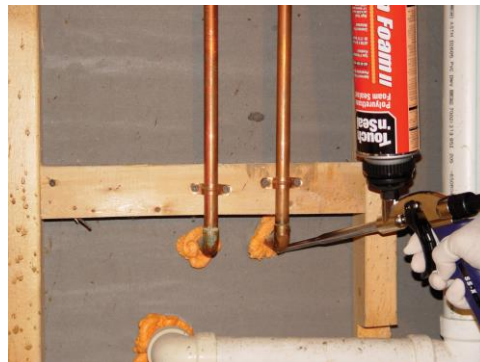
Figure 3 – OCF Dispensing Gun System
